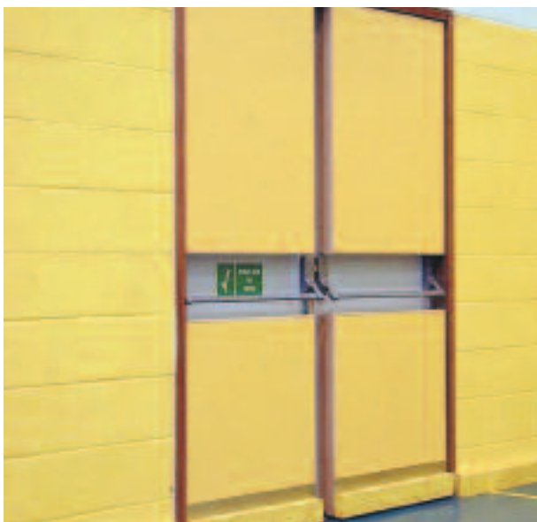
Rebound panels can be fitted above and below panic bolt pressure bars to produce a flush surface.
