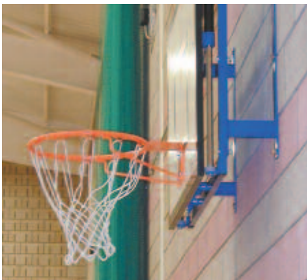
Practice basketball goals on the side of the hall should be height adjustable.
