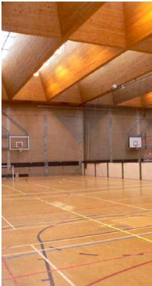
John Wright Sports Centre, heated by warm air heaters.
