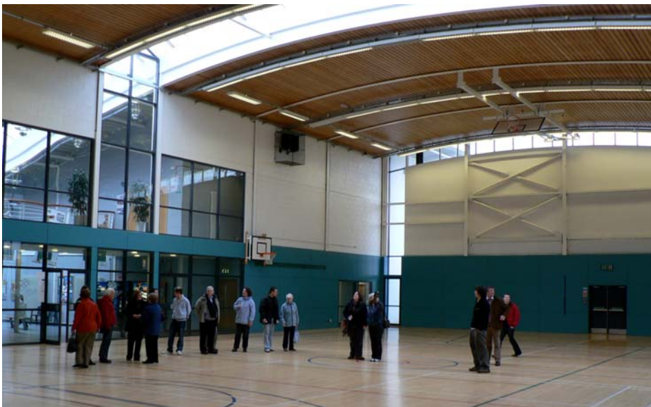
Donald Dewar Sports Hall, Drumchapel, heated by underfloor heating.
