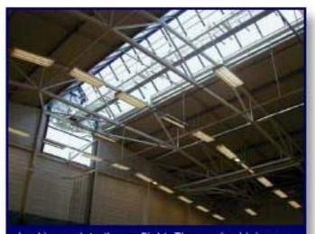
Looking up into the rooflight. The sun is shining on the white painted metalwork. The catwalk adds significant cost to the hall, but is a necessity at these heights, for cleaning and maintenance.
