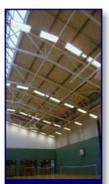
The transition between daylit and artificially lit areas of the hall are helped by the close match between the daylight and fluorescent lighting. Luminaire layout should co-ordinate with the badminton courts. Other sports will then be satisfied too.
