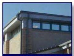
Close up external view of clerestories and eaves overhang. Reflective coating can be seen on the windows.
