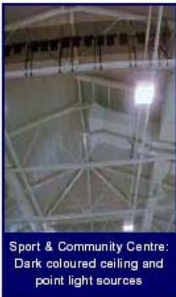
The lighting design needs to consider the colours and reflectances of the hall, and vice versa, so that areas such as ceilings are illuminated correctly. The photo on the left shows the ceiling of a daylit hall, which is grey and is of a low reflectance. The chosen luminaires are capable of providing uplighting, but this facility has not been used here, and even if it were, the poor ceiling reflectance would not help. The ceiling also appears cluttered, which does not help badminton players.
