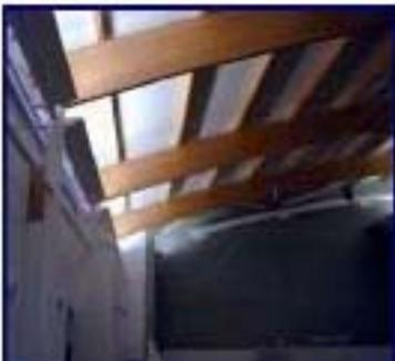
Narrow, hidden clerestories and uplighting to the ceiling have the potential to be successful, but the purlins and dark surfaces cast shadows and create contrast. A player will find it difficult to track a fast moving ball or shuttlecock in these circumstances. The window area is too small to provide sufficient daylighting to have an impact on reducing use of artificial lighting. The uplighting is not the most energy efficient solution, despite its potential benefits.
