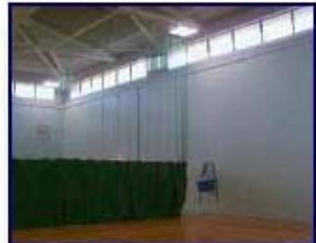
A dark ceiling and dark window frames create poor internal light distribution and risk glare problems. The windows have solar control tint which does reduce the sky brightness. However, with direct sunlight there is little effect and the daylight has little opportunity to spread within the hall due to the poor reflectivity of the ceiling. Artificial lighting is therefore always required.
